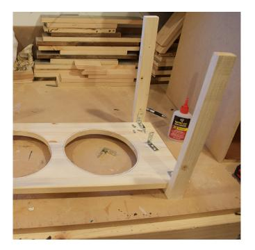
7. Apply RapidFuse to the bottom of the Top Piece and adhere your legs to the main board. Use a drill to screw the corner braces to the bottom of the main board to the legs. This will add strength to the bowl stand and ensure the weight of your bowls will not break the stand.
